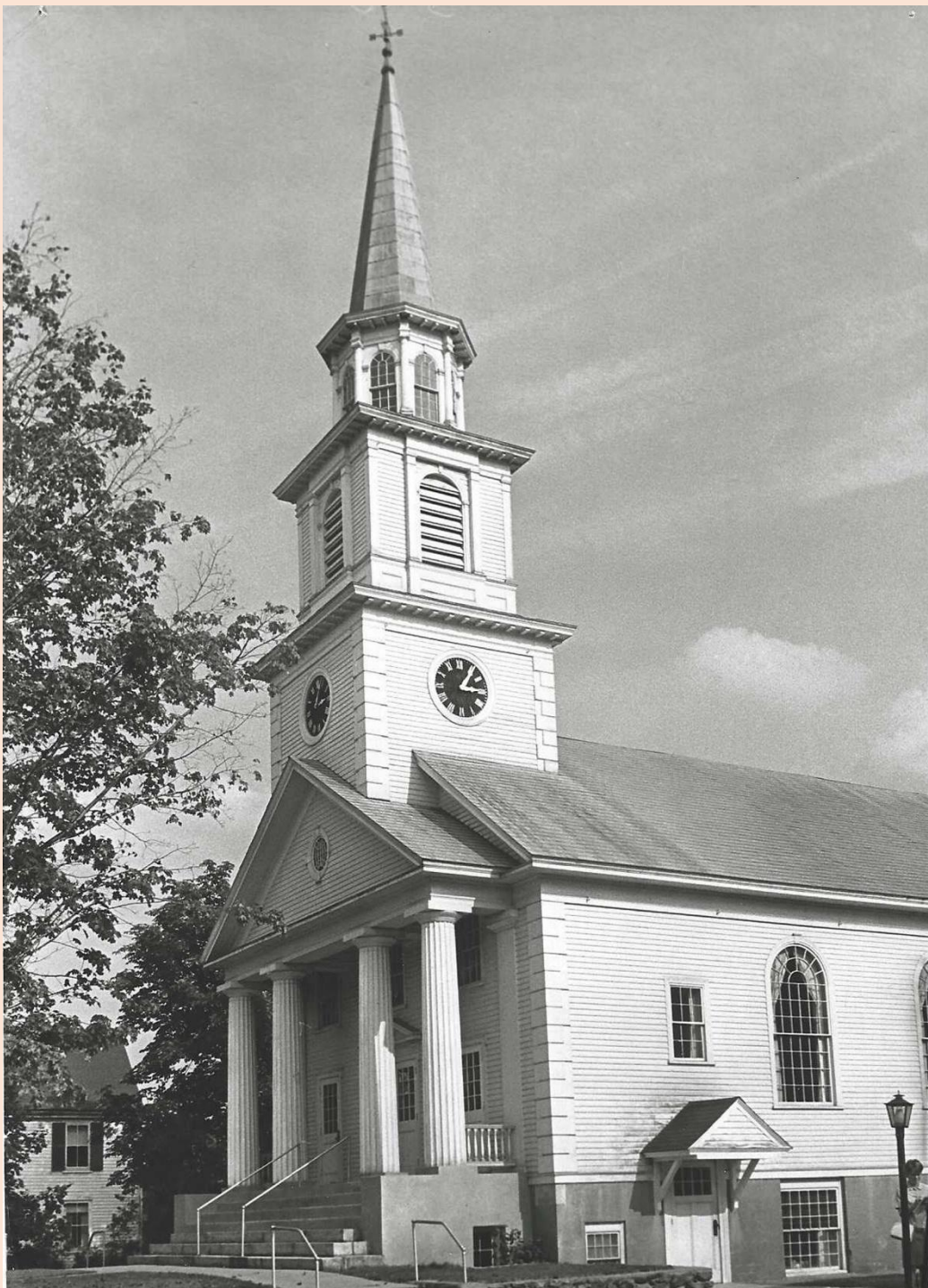
FIRST CONGREGATIONAL CHURCH Dedicated November 6, 1927 Boylston, Massachusetts
